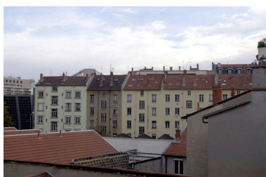
Elévation postérieure Phot. Maryannick Chalabi IVR82_20086900643NUCA
