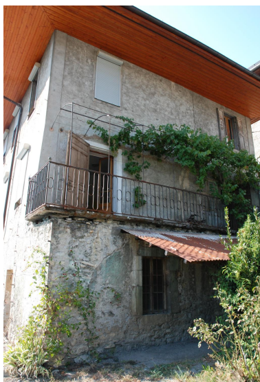
Elévation est. Phot. Caroline Guibaud IVR84_20247301562NUCA
