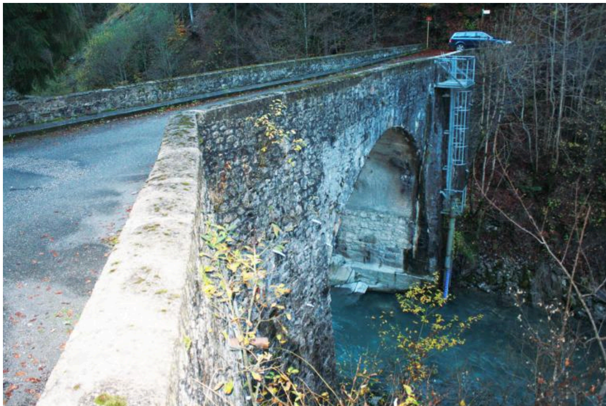
Pont de Couvaloup, face aval
