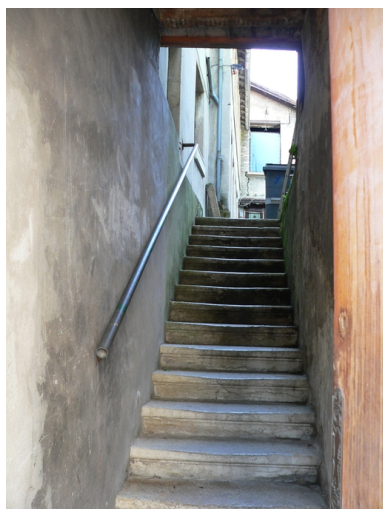
Escalier Phot. Isabelle Dupuis IVR82_20093800477NUCA
