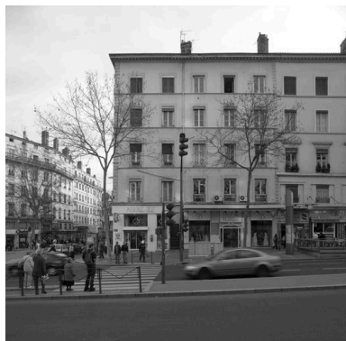
Elévation, cours Gambetta Phot. Eric Dessert IVR82_20056900576NUC
