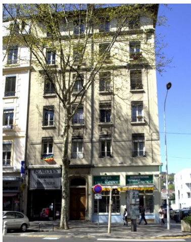
Elévation principale Phot. Maryannick Chalabi IVR82_20036900361NUCA
