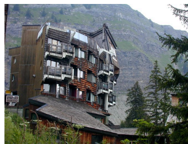
Elévation sud Phot. Jean-François Lyon-Caen, Phot. C. Salomon-Pelen IVR82_20087401104NUCA
