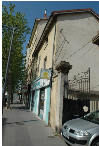
Façade principale, vue est. Phot. Nadine Halitim-Dubois IVR82_20096901779NUCA
