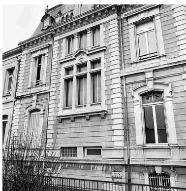
Façade nord Phot. Martial Couderette IVR82_20042600039X
