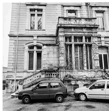
Entrée principale Phot. Martial Couderette IVR82_20042600044X
