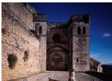
Façade. Phot. Eric Dessert IVR82_20002600985PA
