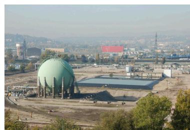
Rhône-Poulenc usine 2009 (BML : P1236 001 0169) Phot. Jules Sylvestre IVR84_20256900077NUCA
