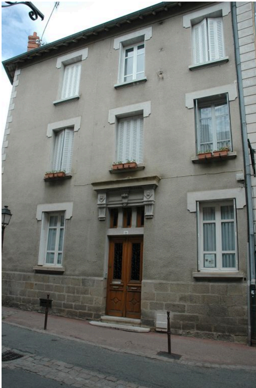
Elévation principale, rue Martin-Bernard.
