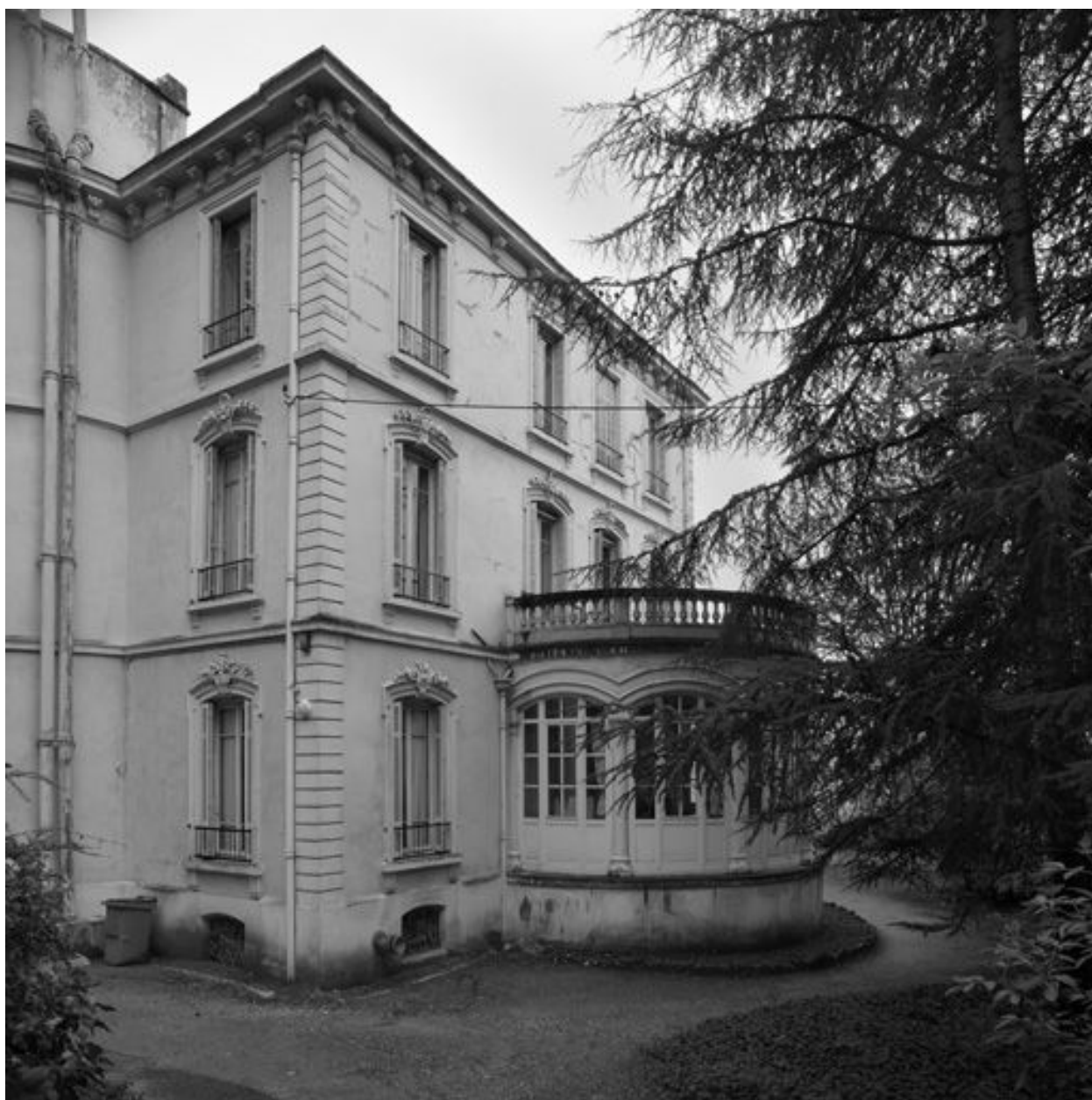
Logis, façade sud
