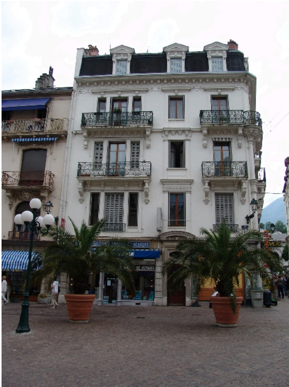
Façade, place Carnot
