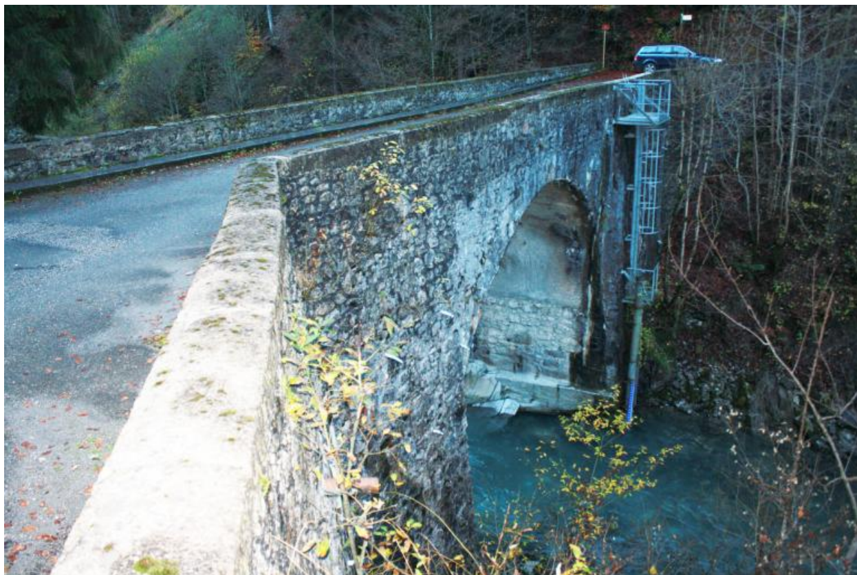
Pont de Couvaloup, face aval
