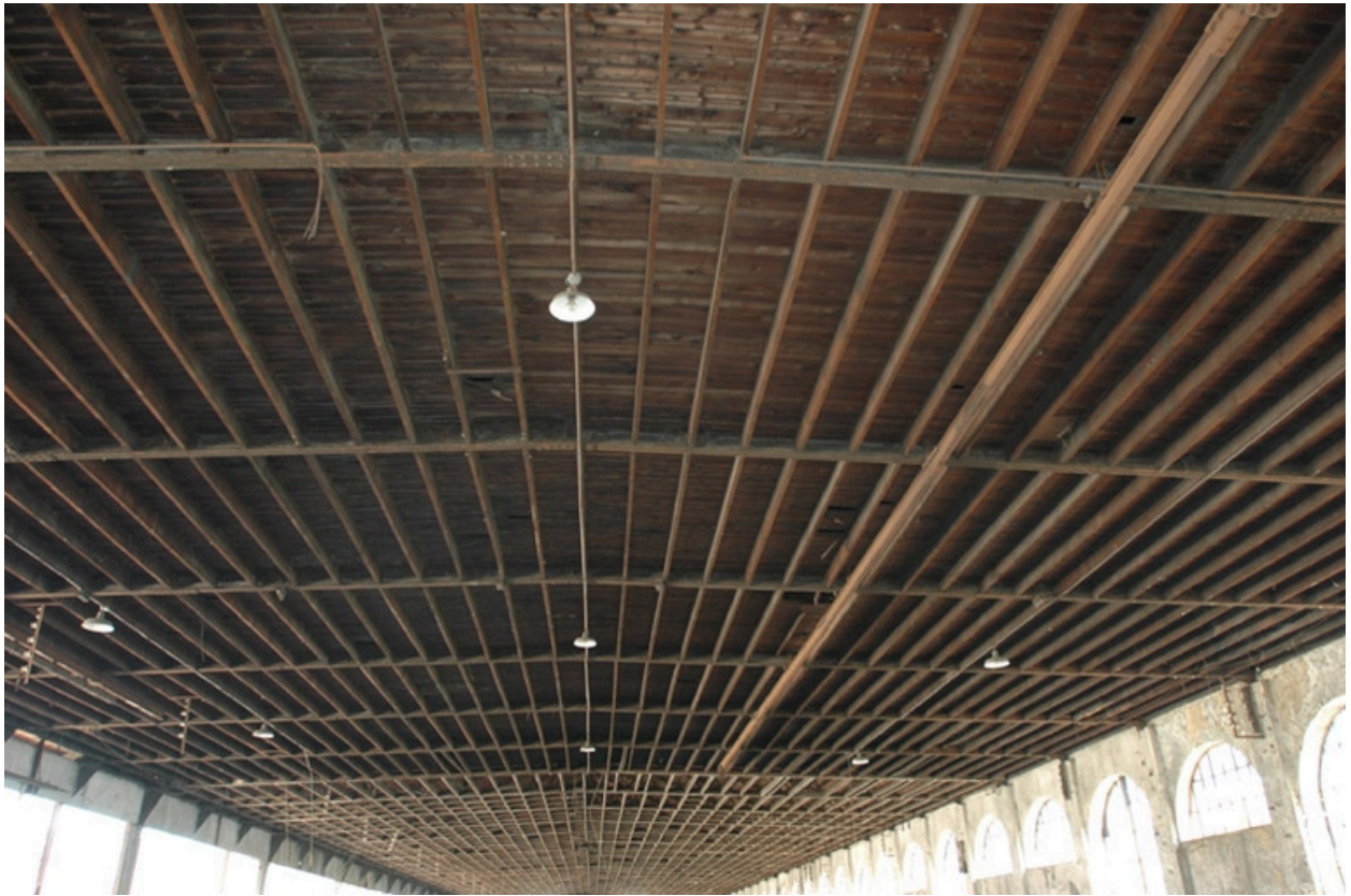
Charpente grande halle
