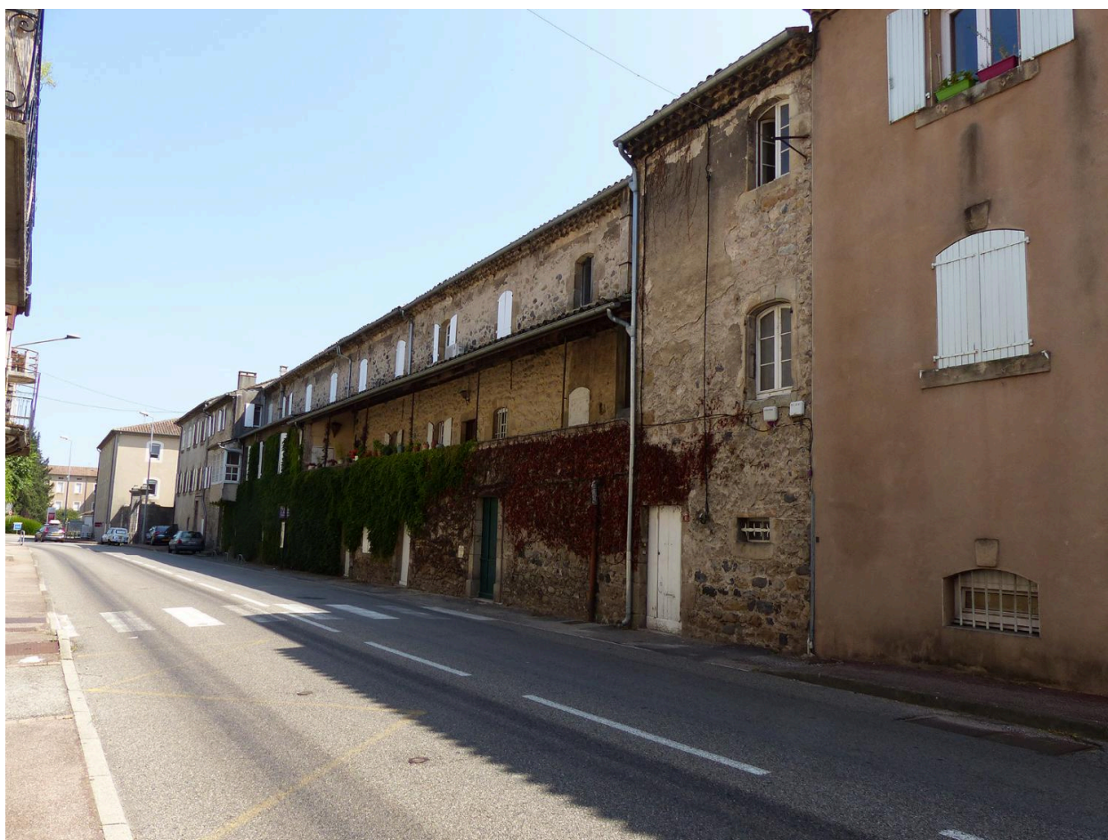
Manufacture Royale Deydier façade principale
