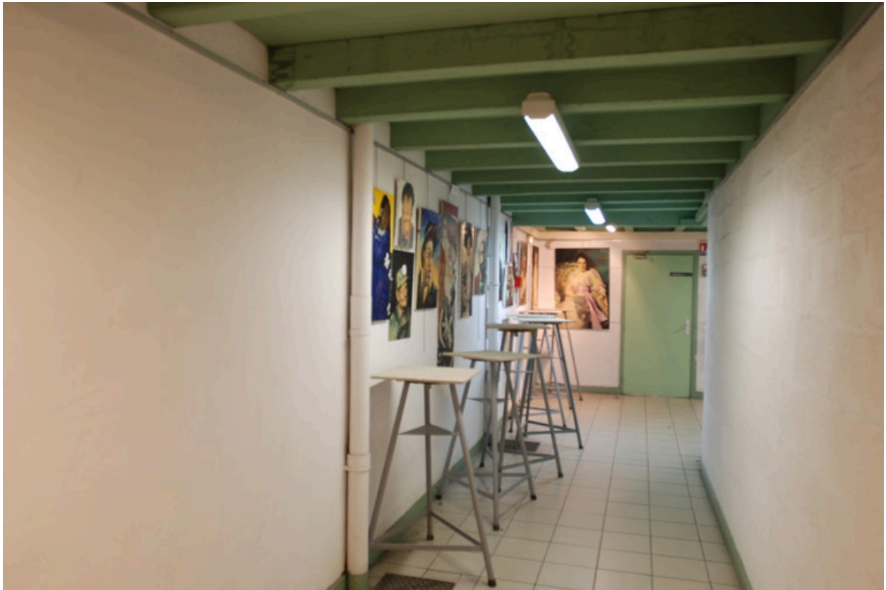
Couloir de distribution
