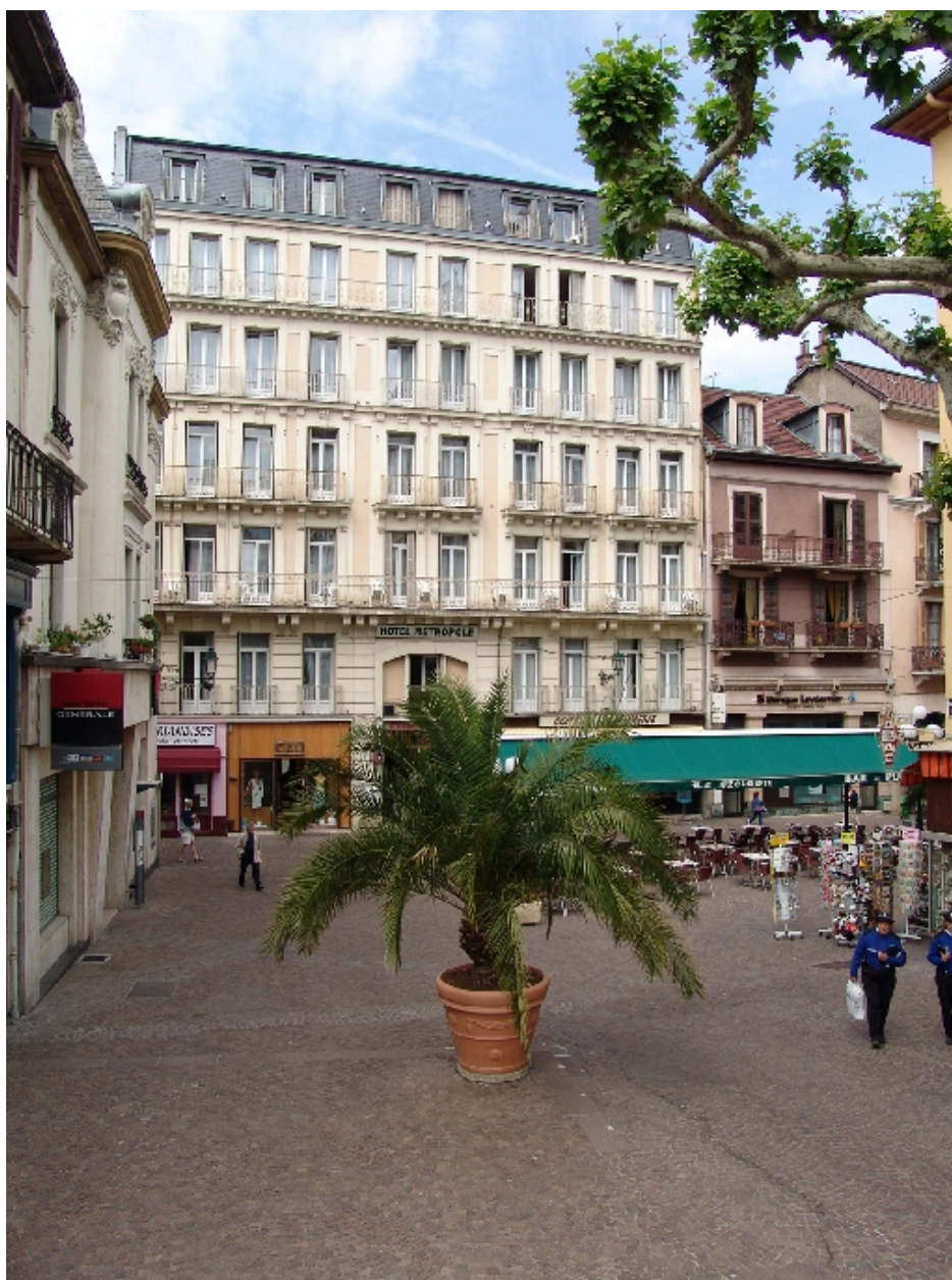
Façade place Carnot
