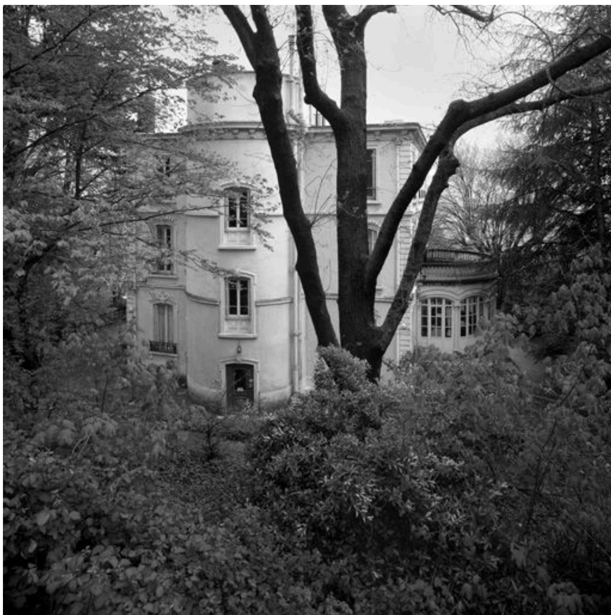
Logis, façade nord
