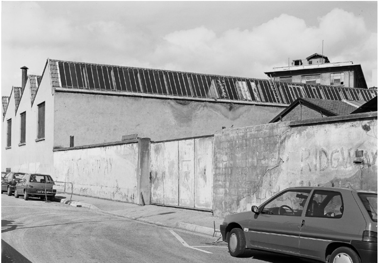
Vue est, sheds.
