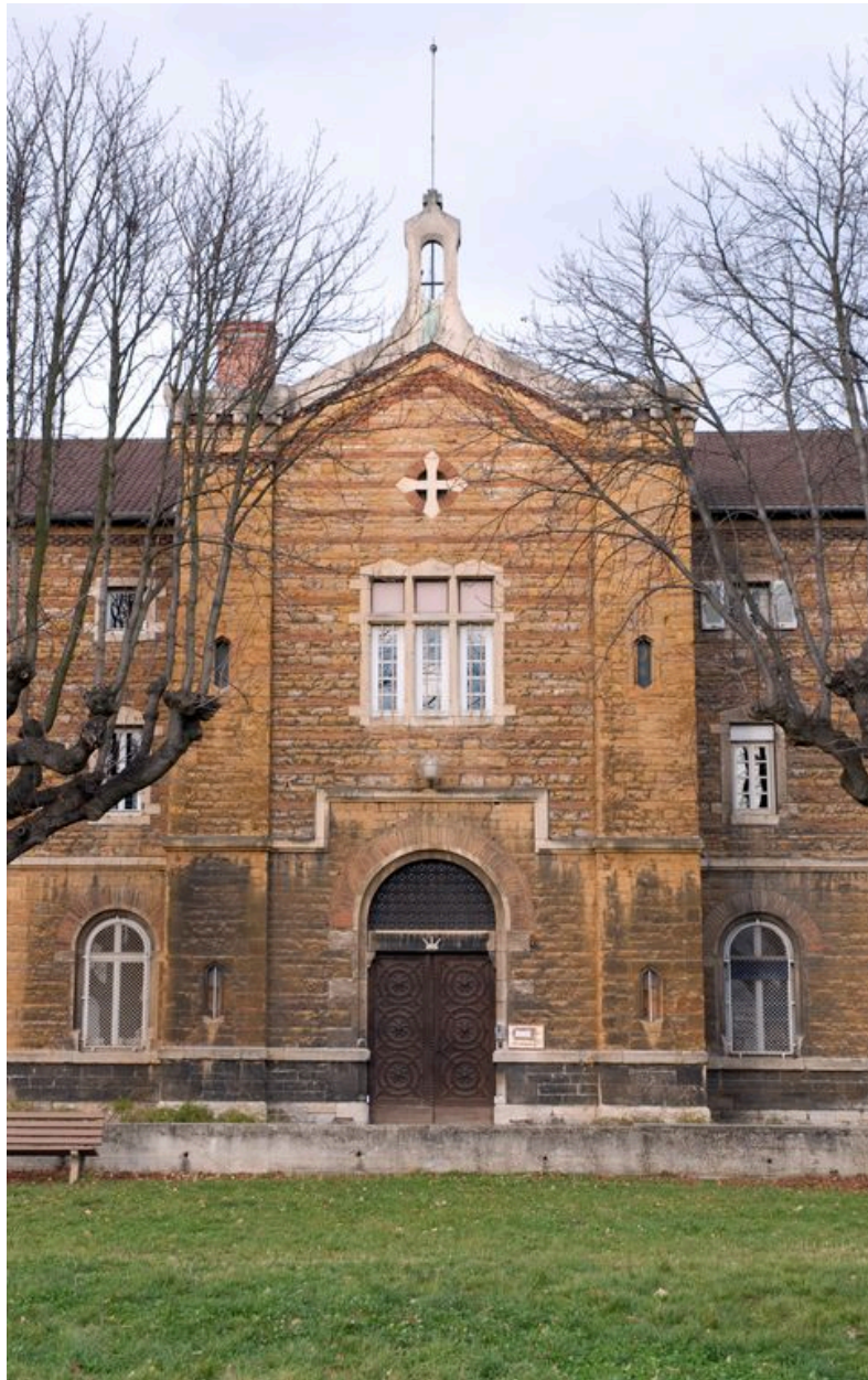
Elévation principale, avant-corps central
