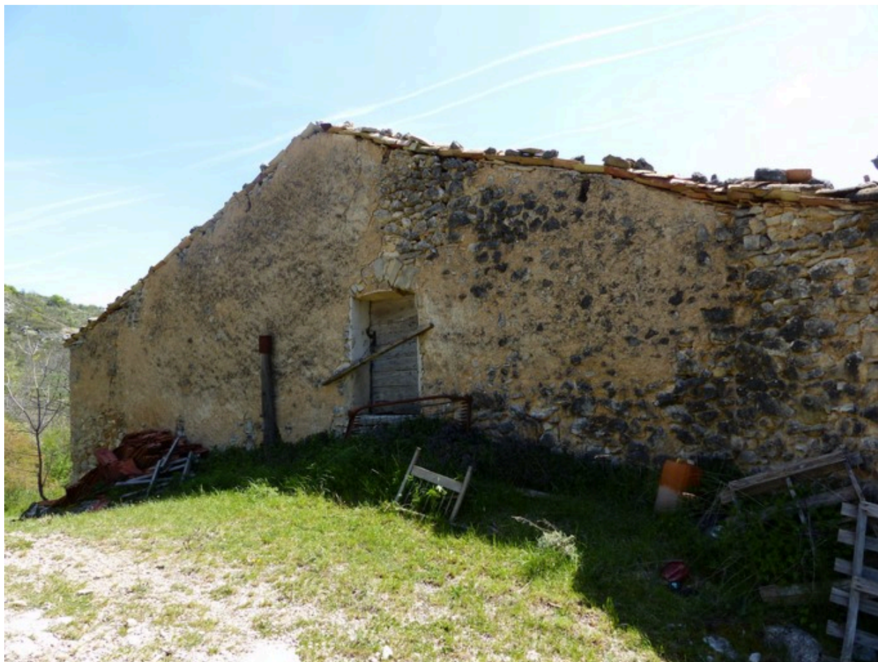
Ensemble oriental. Pignon nord.
